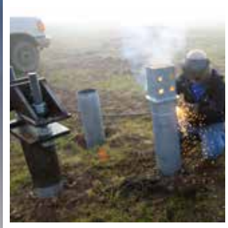
Pier top removal by plasma torch
