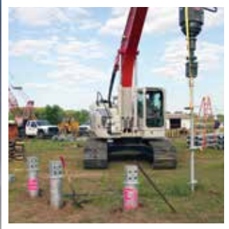
Helical pier installation
