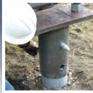
Adapter caps secured on piers
