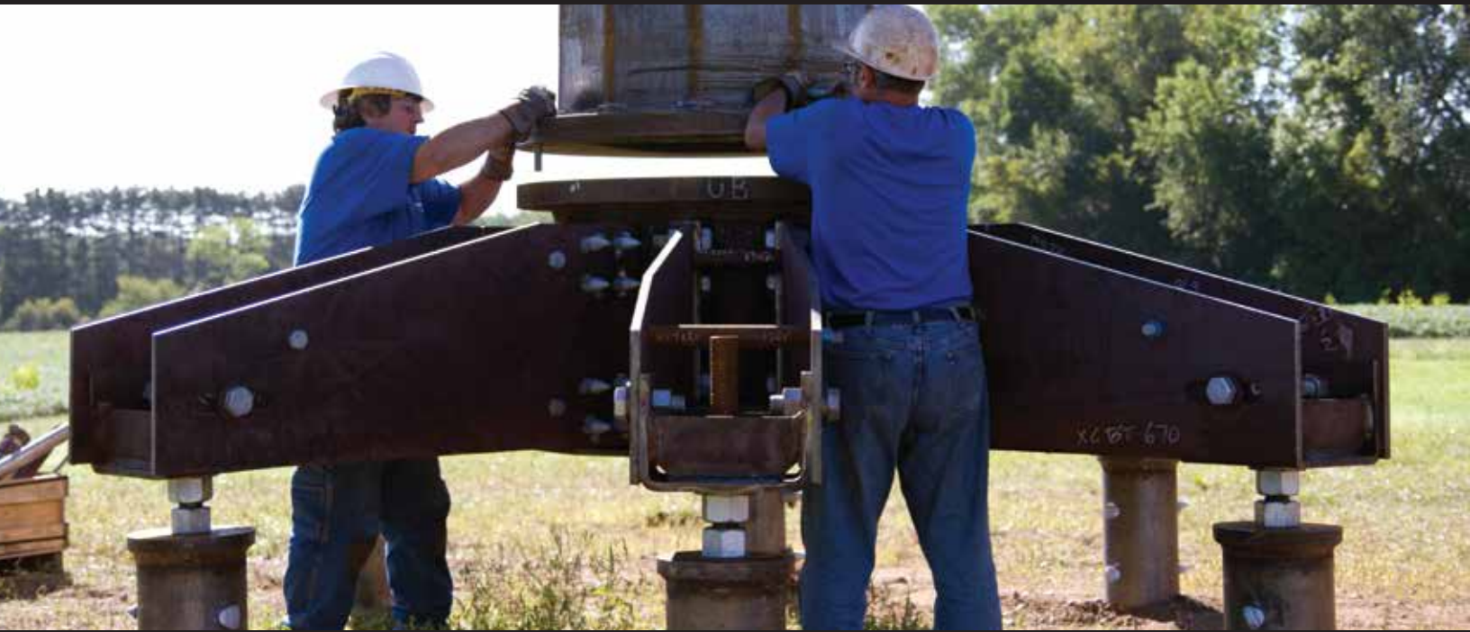
Pier top removal by plasma torch
