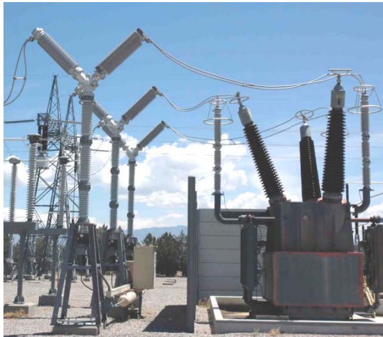
Fig. 4. Shunt reactor switched with a SF 6 breaker
