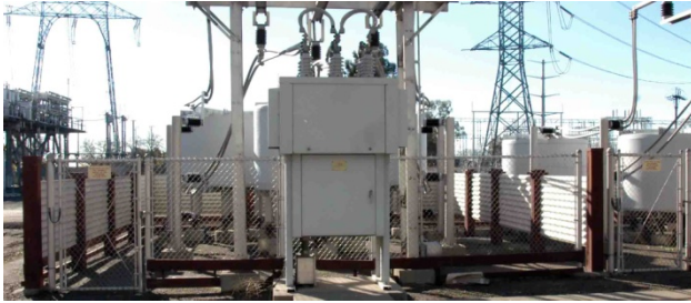
Fig. 5. Air-core dry type shunt reactors switched with a vacuum device
