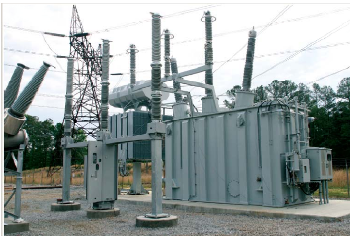
Fig. 6. 230 kV Special purpose shunt reactor switch
